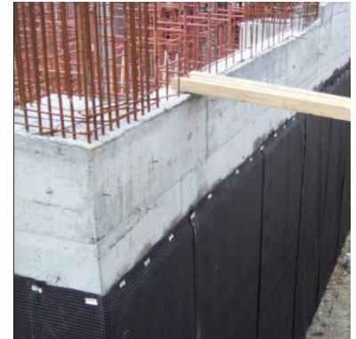
Protection of the Coating
